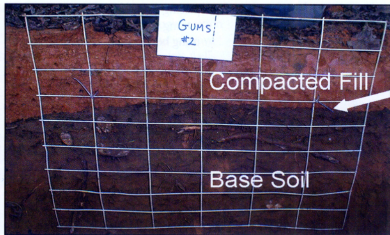
Figure 6. Moisture in the root zone may be affected by fill soils. Here, the underlying soil is relatively dry compared to the overlying fill. The difference in soil texture between the fill and base soil might have restricted water movement into the base soil. In some cases, rainfall and water applications may not be sufficient to percolate through the fill and wet the base soil.
